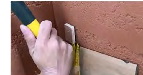
12. After it is completely dry, pull out the air nails
