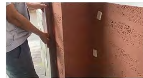
4. Measure the construction size with a ruler
