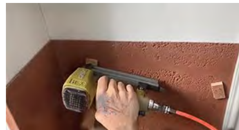
3. Fit it with air nails
