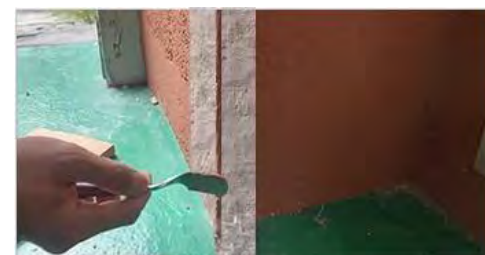
9. Use a scraper to smooth the caulk
