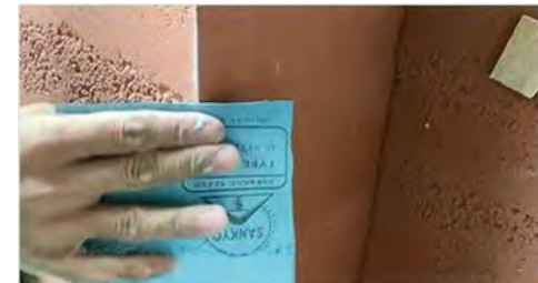
10. Grind the edges and corners
