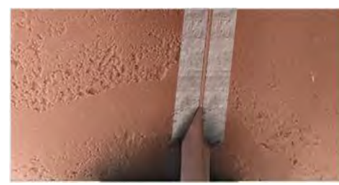
7. Fill the internal corners with caulk
